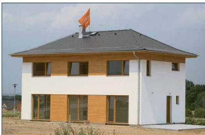
Ventilation of roof frame by combination of ridge ventilation and cowl vents.
