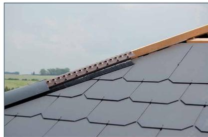
The size of exit hole with ridge ventilation is 100 cm<sup>2</sup> /m. Air space is 1 cm/m.
