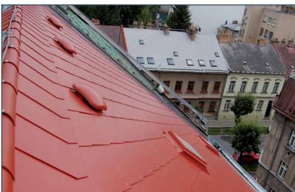
Ventilation of roof frame with plastic ventilation terminals.
